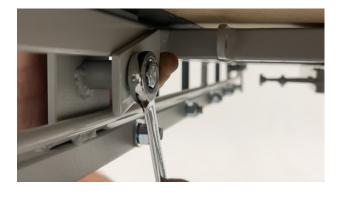
Once in position fit clamp plates and tighten bolts with 16mm spanner.
